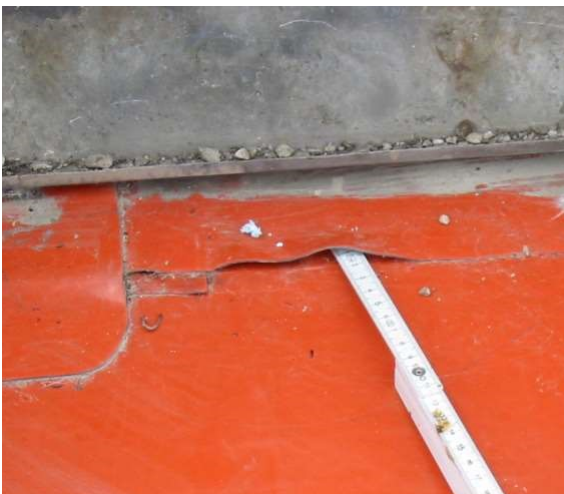
Examples of open seams after 13 and 15 years of exposure time.
