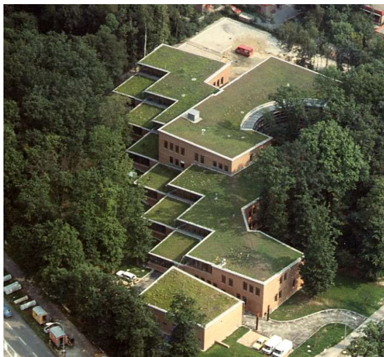
Object example, year of construction 1987 , (now 30 Years), PVC-membrane, thickness: 2,4 mm,
