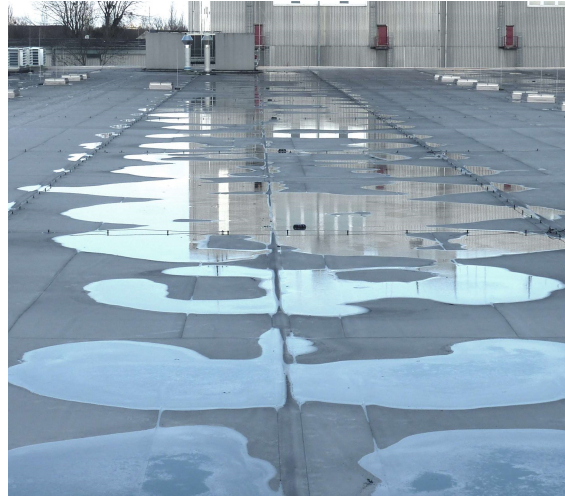
Example of: TPO-membrane, thickness 1.8 mm, with temporary water ponding.
