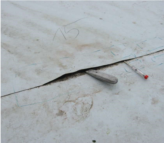
Examples of open seams after 13 and 15 years of exposure time.
