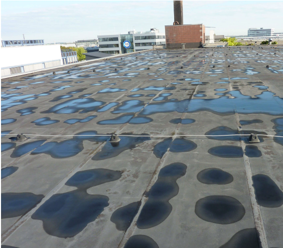
Example of: PVC-membrane, thickness 1.5 mm, with temporary water ponding.
